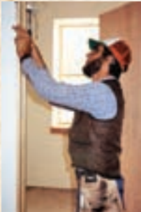
Armand Martin is shown working on the office rehab in 1991.
